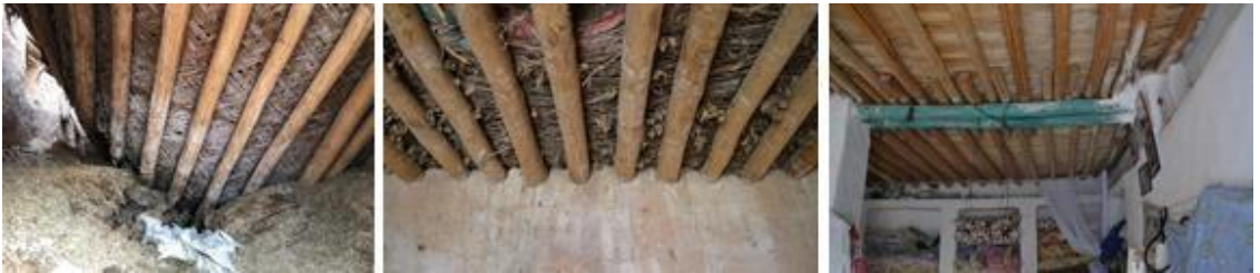
Figure 7. Beams and interlayers, 2019.
