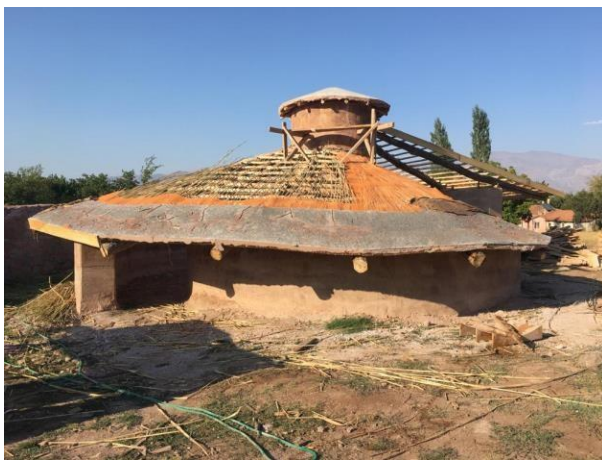
Figure 18. Layers visible during roofing, 31 August 2021
