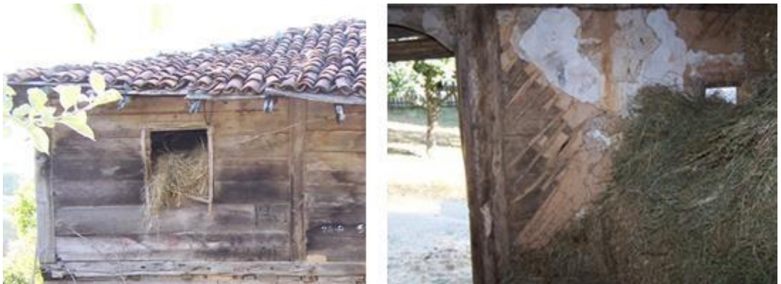
Figure 8. Views of the timber masonry wall from the outside and inside
