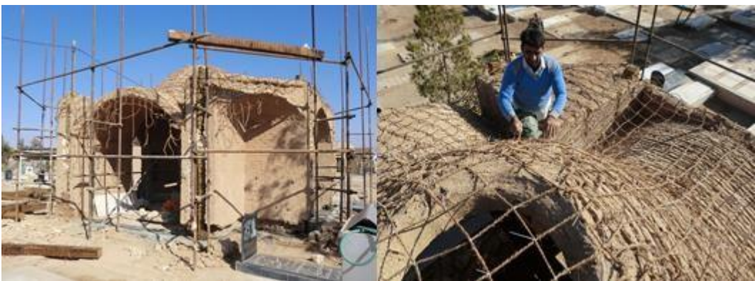
Figure 13. Removing the old dome and rebuilding the new one
