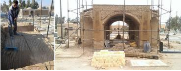
Figure 11. Removing the hollow spandrels and reassembling them
