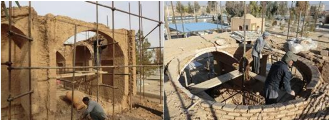
Figure 12. Removing the old dome and rebuilding the new one
