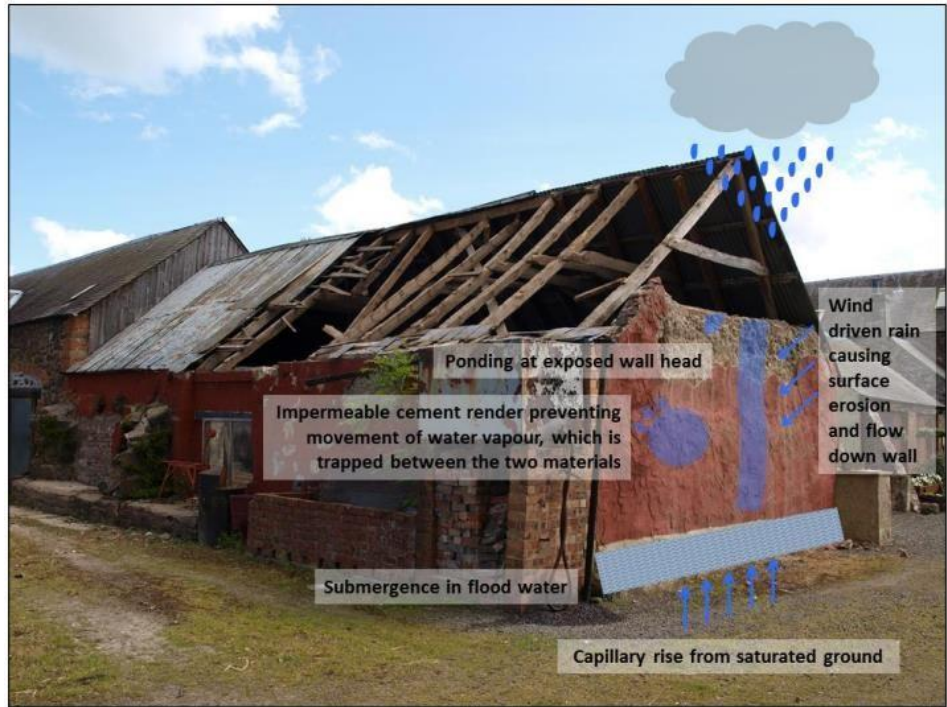
Figure 3. Typical water-ingress problems [22]
