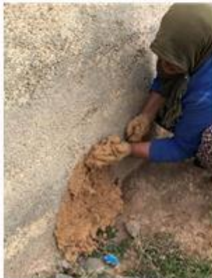
4. The mortar is adhered to Wall to the plastered.
