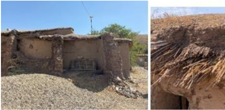
Figure 15. Collapsed roof and destroyed walls, greening of earthen roof (2021)
