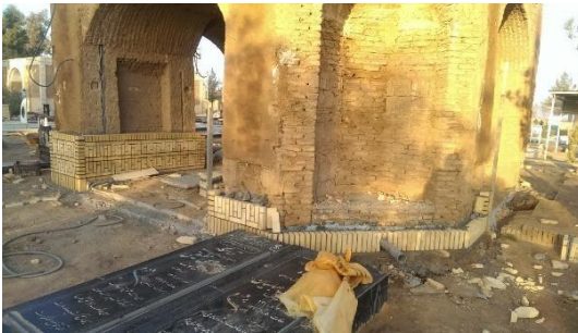
Figure 15. Executing plinth inside and outside the tomb
