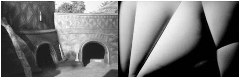
Figure 5. Houses constructed with wet sculpting technique in Ghana (left), a ceiling design to molded earth which can be constructed pouring mineral loam in formwork of textile stressed by cables (Minke, 2006).
