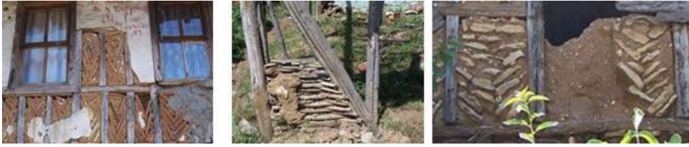
Figure 7. The use of adobe mortar between the stone, brick, wattle, and daub filling on the timber-framed skeleton wall.
