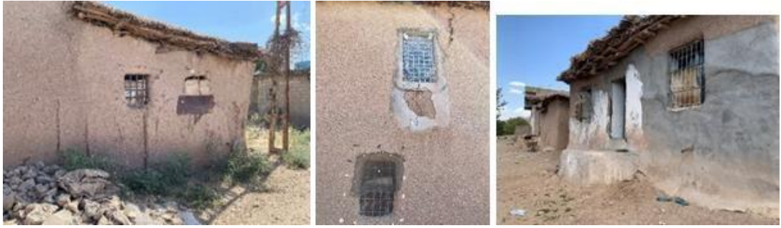
Figure 17. Fractures and cracks on the walls, replacing windows and doors with PVC and metal materials, cement-based plaster application (2021)
