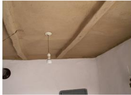
Figure 11. Adobe plaster on a wall; Figure 12. Adobe plaster on the ceiling
