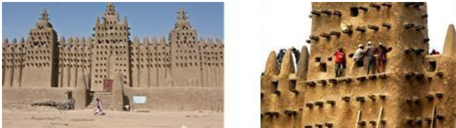
Figure 13. The platform on which the mosque is placed [URL 18]; Figure 14. Wooden overhangs on the facade [URL-19]
