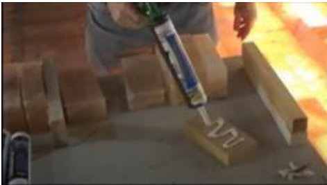
Figure 18 & Figure 19. Using strong glue specified for Himalayan salt bricks.
