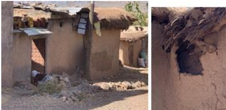
Figure 16. Covering the collapsed roof with metal sheets, adobe plaster openings, cracks, ruptures and spills (2021)
