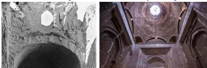
Figure 5. Sholdred arches in kooh-e-khaje[8](left), Se Gonbad tomb (right)
