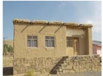
Figure 7. Mortar preparation pool; Figure 8. Adobe production using the field; Figure 9. Adobe wall home, loadbearing wall system
