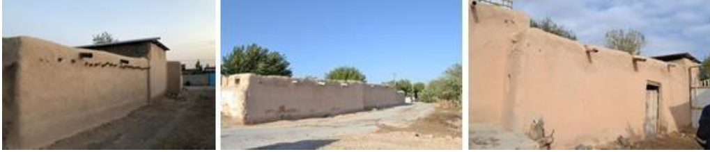
Figure 6. Facades plastered with mud plaster, 2019.
