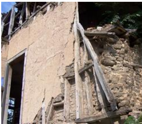
Figure 5. Filling adobe blocks on a timber-framed skeleton wall; Figure 6. Filling adobe blocks with brick blocks on a timber-framed skeleton wall
