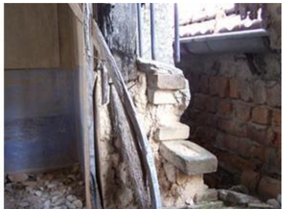
Figure 5. Filling adobe blocks on a timber-framed skeleton wall; Figure 6. Filling adobe blocks with brick blocks on a timber-framed skeleton wall
