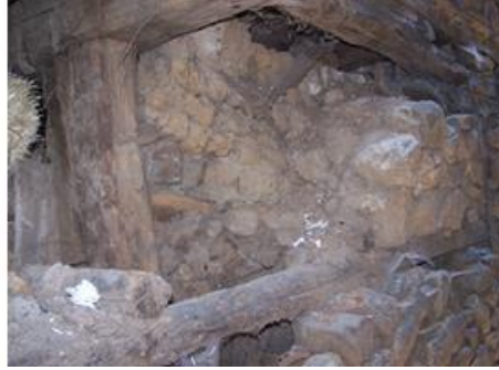
Figure 3. Adobe block - brick layered masonry application (Brick outside, use of mudbrick inside); Figure 4. Adobe block - brick layered masonry application (Brick outside, use of mud-brick inside)
