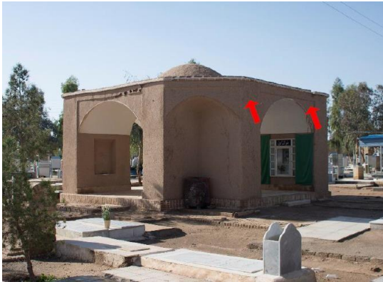
Figure 5. Possibility of falling off the eaves on the north
