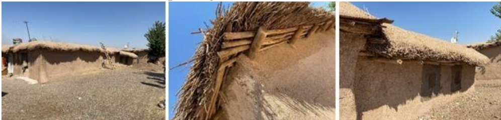
Figure 11. Flat earthen roof (2021)
