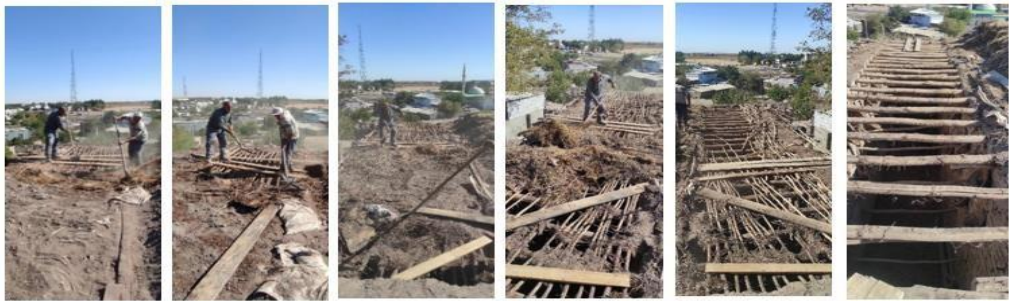
Figure 14. Dismantling of the roof
