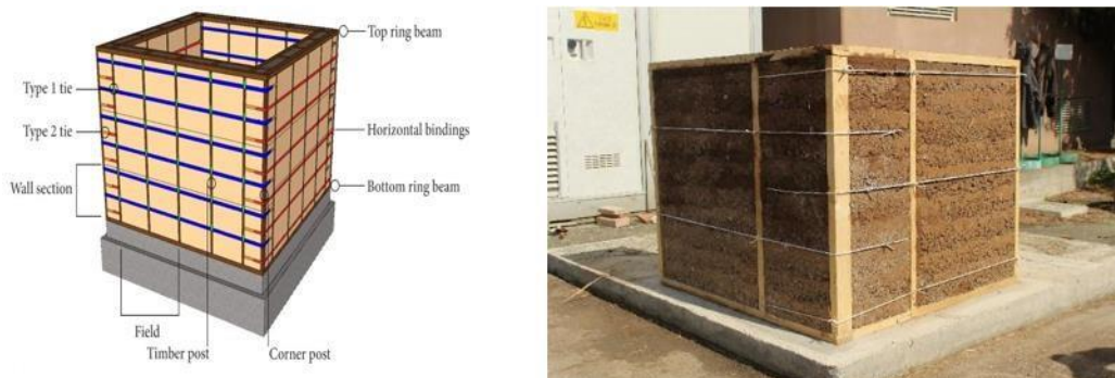
Figure 1. Three-dimensional reconstruction of the reinforcement system (on the left) and prototype wall for the validation of the constructive process (on the right).
