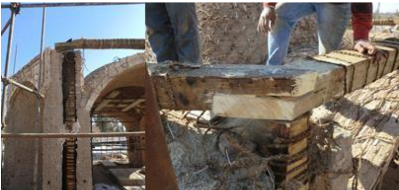
Figure 10. Embedding the posts in the grooves and jointing them to the beams
