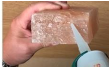
Figure 18 & Figure 19. Using strong glue specified for Himalayan salt bricks.
