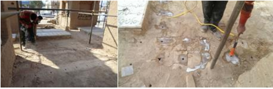
Figure 14. Making the holes and injecting the poison
