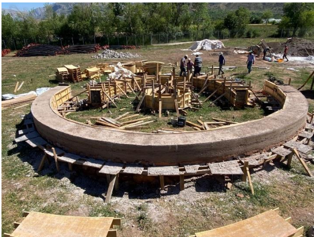
Figure 10. The first 60 cm of the two main earth walls were built., 10 June 2021
