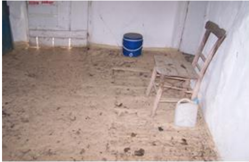
Figure 10. Adobe coating on timber flooring at the mezzanine level
