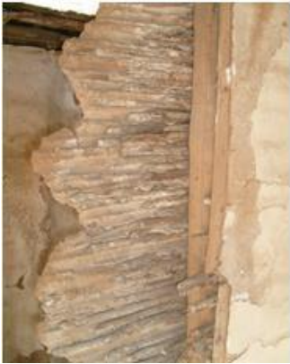
Figure 13. The Baghdadi wall is being filled and plastered with adobe mortar
