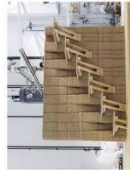
Figure 4: 3D printing adobe wall with built-in staircase
