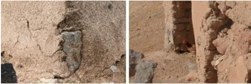
Figure 4. Stone foundations in traditional buildings, 2019.
