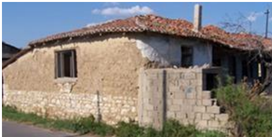
Figure 2. Adobe masonry wall examples
