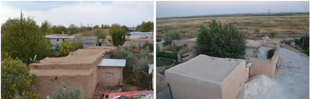
Figure 8. Traditional flat earthen roofs, 2019.
