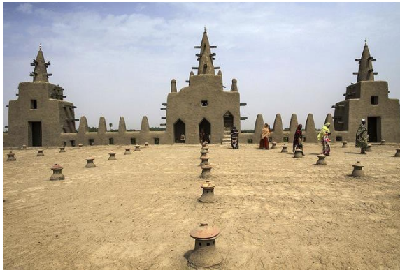
Figure 11. Ventilation chimneys on the roof [URL 10]
