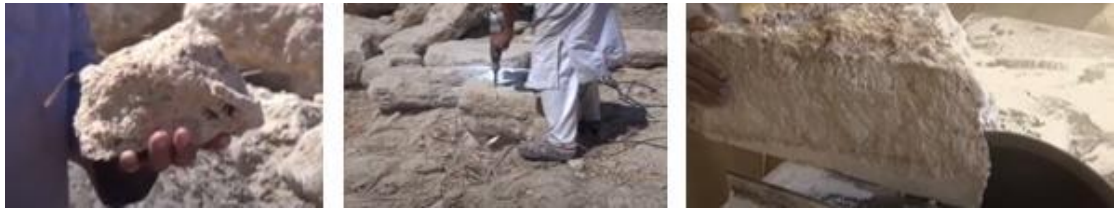
Figure 6. The Salt rocks after extracting and preparing for cutting and cleaning, Siwa Oasis-Egypt (author, R. Elborgy); Figure 7 & Figure 8. Cutting and shaping the salt rocks in forming to use, Siwa Oasis-Egypt (URL1, video)
