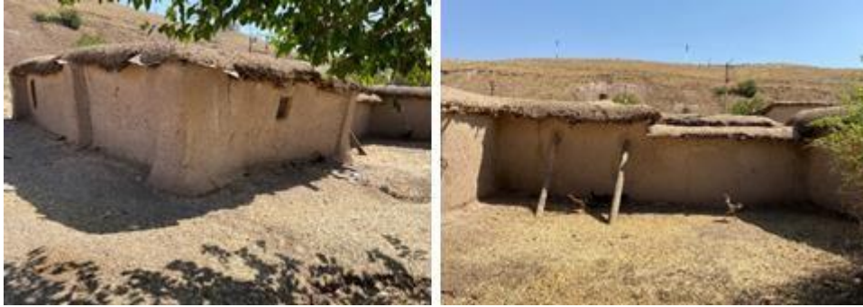
Figure 14. Structural problems, inability of walls to carry the roof load (2021)
