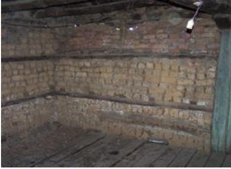
Figure 3. Adobe block - brick layered masonry application (Brick outside, use of mudbrick inside); Figure 4. Adobe block - brick layered masonry application (Brick outside, use of mud-brick inside)
