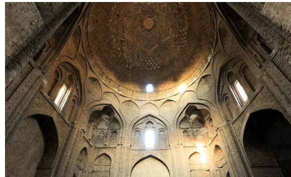
Figure 6. Patkaneh under the north dome of Jameh Mosque of Isfahan
