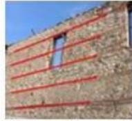
The use of beams in masonry buildings [2]
