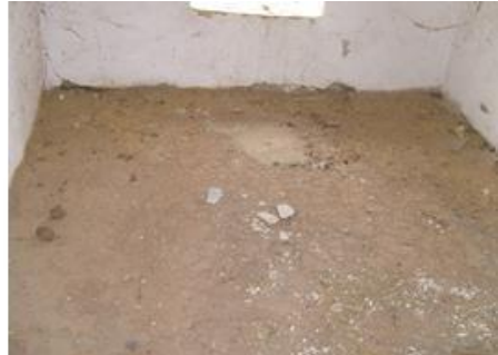
Figure 10. Adobe coating on timber flooring at the mezzanine level
