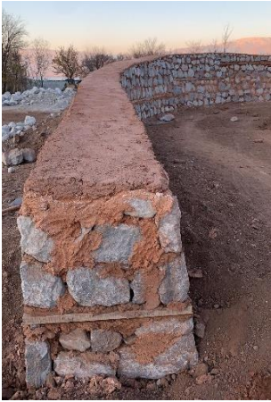
Figure 9. Retaining wall as a wind barrier with horizontal wooden beam inside, December 2019
