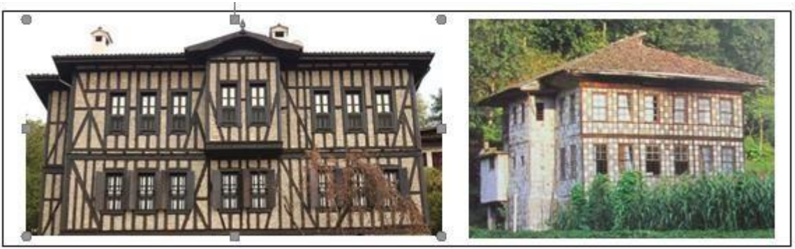
Figure 10. Cross-linked texture on wall surface suitable for adobe material with dense interspaces [25]; Figure 11. Wooden frame system with square partitions “Göz-Dolma” [26]
