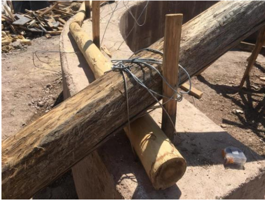
Figure 15. Poplar purlins and pillow wooden beams joint detail, 27 June 2021
