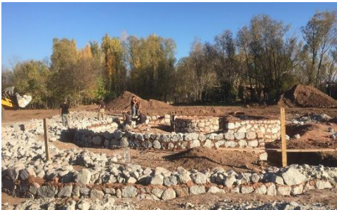
Figure 8. Stone foundation upper level is 20 cm above ground, November 2019
