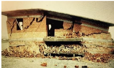
Figure 10. Diagonal cracks, no earthquake precautions
