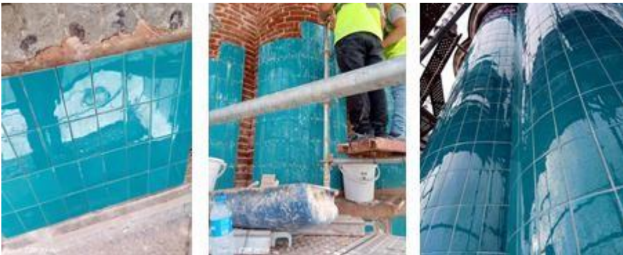
Figure 20. The tiles are applied with khorasan mortar (Resource: Personal Archive); Figure 21. The tiles are applied on the bricks (Resource: Personal Archive); Figure 22. The tile application is finished (Resource: Personal Archive)
