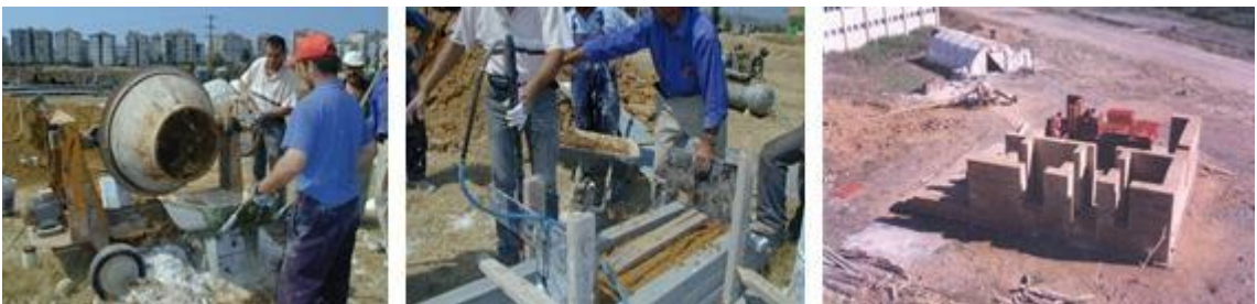
Figure 14. Concrete mixer for mortar: 100kg earth, 10kg gypsum, 5kg lime and water; Figure 15. Ramming mixed mortar in to the wall-form with Compactor; Figure 16. TUBİTAK 662- research building -rammed into the form.
